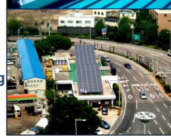
Busan city Highway office 35kW
