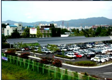
Korail Office Building 90kW
