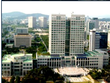
Daejeon City Hall 20kW
